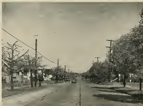
10TH AVENUE, EAST OF ALMA STREET
